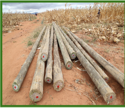
Power poles being prepared and installed for the borehole connections
